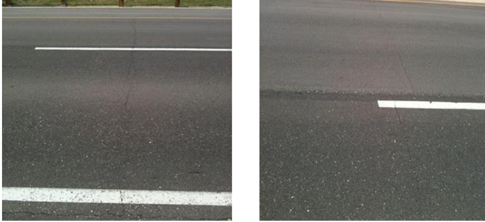
Figure 13 Survey on a project one year after construction (IA-13)
