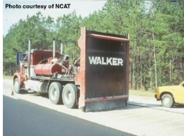
Figure 3 Crack-and-seat
