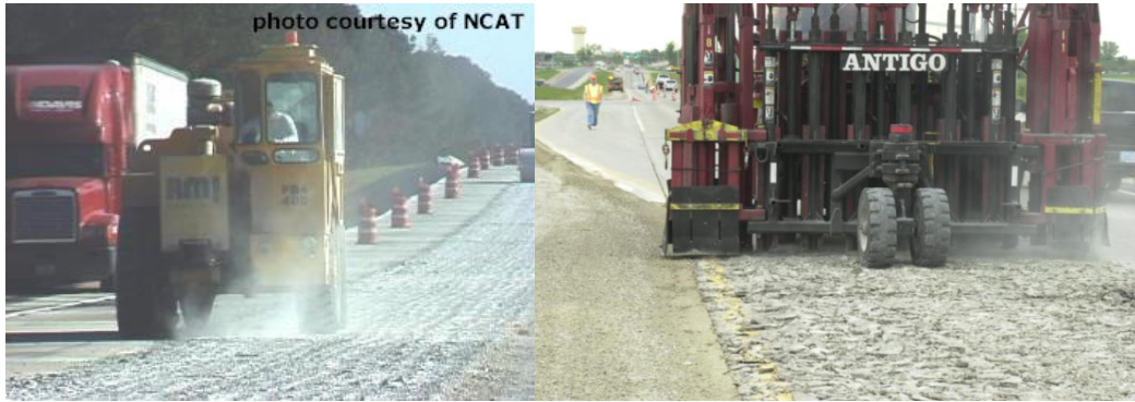
Figure 4 Rubblization: Resonant Pavement Breaker (left) and Multi-Head Breaker (right)
